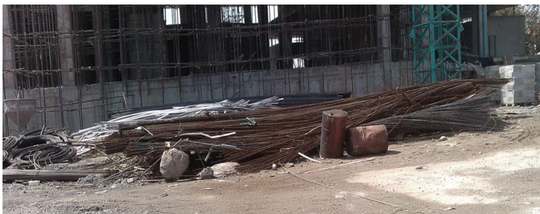
Figure 4.18 Placing of steel rebar in local office building construction project
