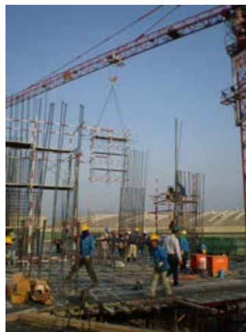
Figure 4.7 Prevention against falling objects from crane operation
