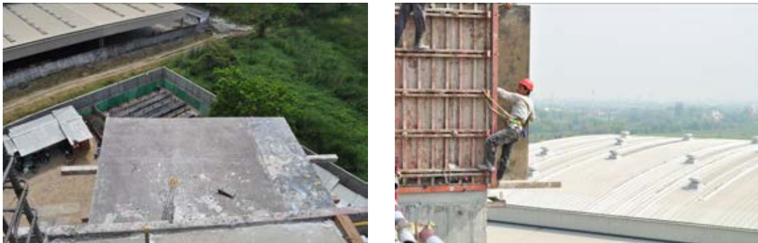
Figure 4.9(a) and (b) Working platform preparation
