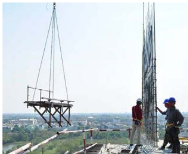
Figure 4.11 Platform installation
