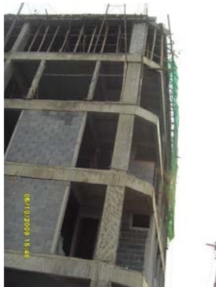
Figure 4.4 Prevention against falling objects from building perimeter
