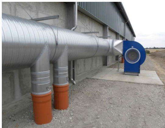
Figure 12 Example of fan ventilation method for warehouse
