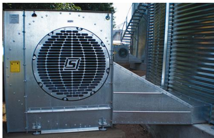
Figure 11 Example of fan ventilation method for silo
