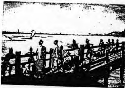
Picture1 U Bein Bridge in Amarapura
