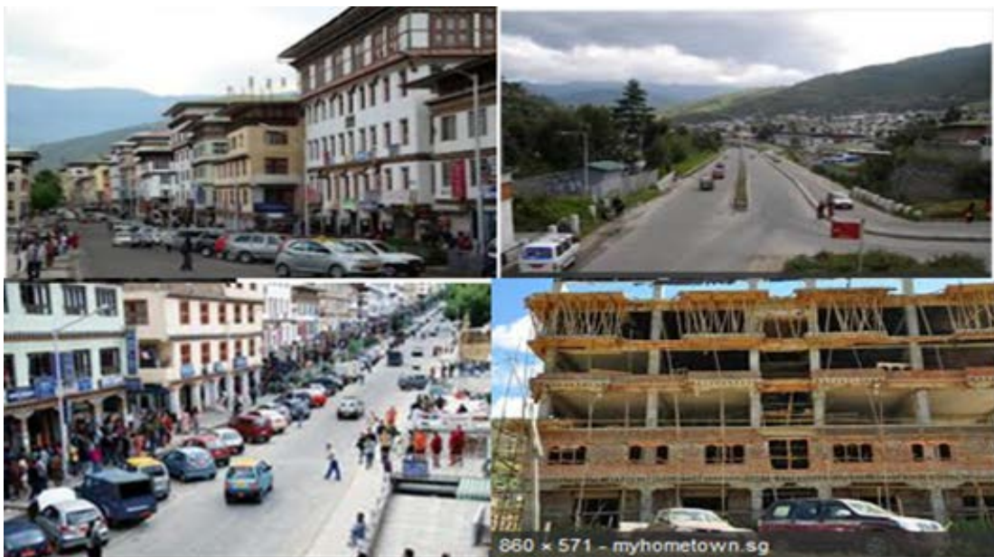
Figure 4-2 The construction in capital city
