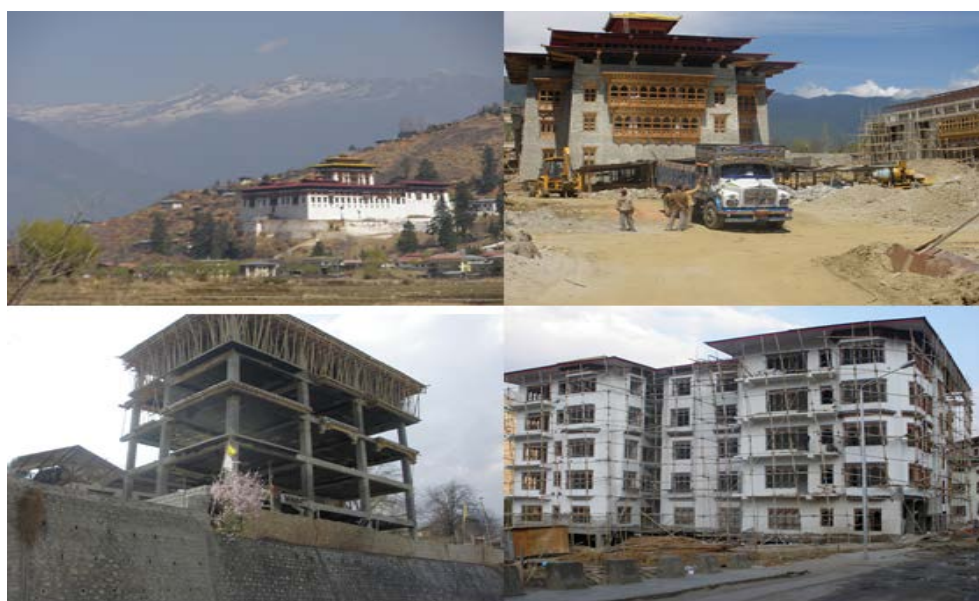
Figure 4-6 Contemporary public construction projects in Thimphu and Paro.
