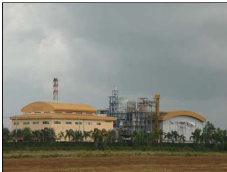
Photograph 11 Decha 7.5 MW biomass power plant in Suphanburi province
