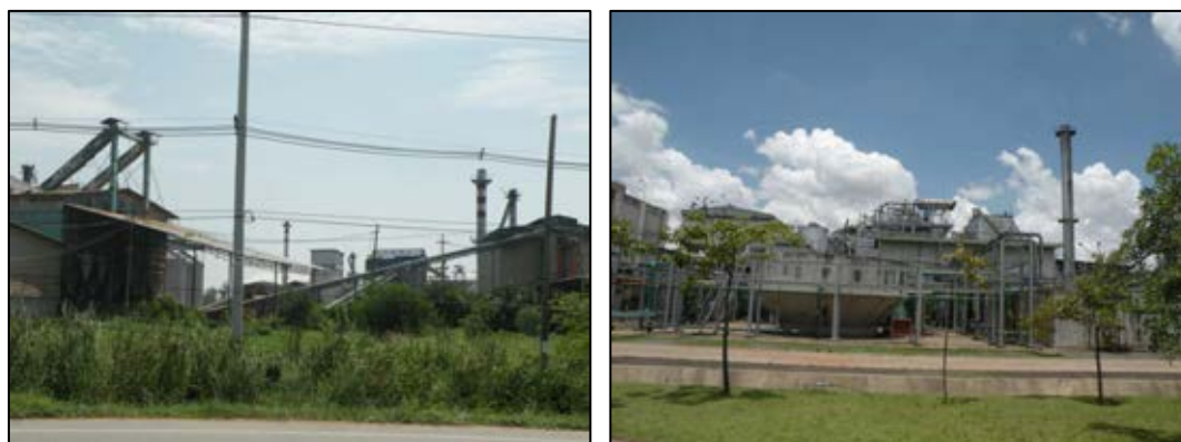
Photograph 1 (Left) Buasommaï 6.4 MW and 9.9 MW biomass power plants Photograph 2 (Right) Roi-Et Green 9.9 MW biomass power plant
