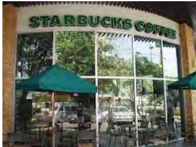
Figure 2.7 First Starbucks in Thailand, Central Chidlom Branch
