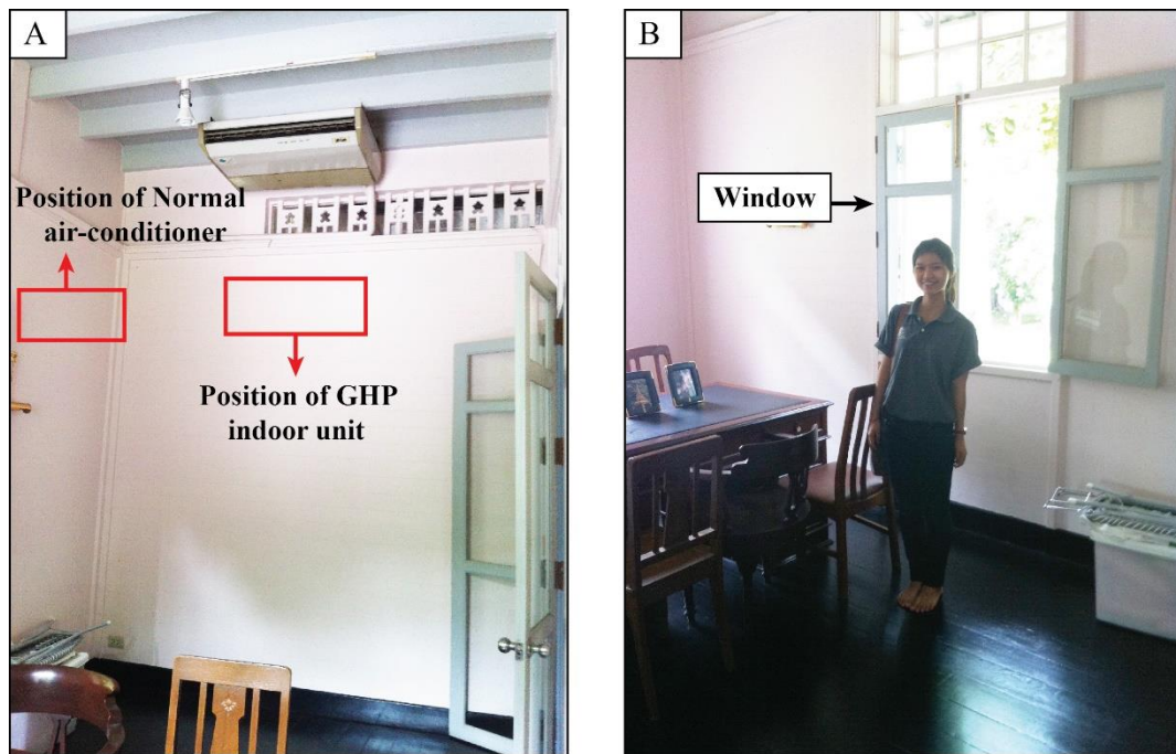
Figure 2.13 Experimental room at the second floor of Parot Racha building with 2.84 meters-wide, 4.74 meters-long and 3.50 meters-high. (A) Position for installing GHP indoor unit and Normal air-conditioner (AC) indoor unit (B) Window of back side of the building (Miss Sasimook Chokchai, tall 160 meters).
