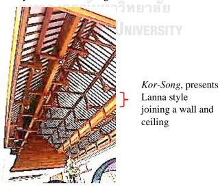
Figure 55:The roof structure.
