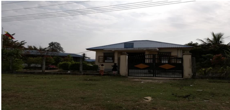
Figure 3.10 This photo shows Nam Jim's village health care centre built by the government. (Photograph by researcher, 11 September 2017).
