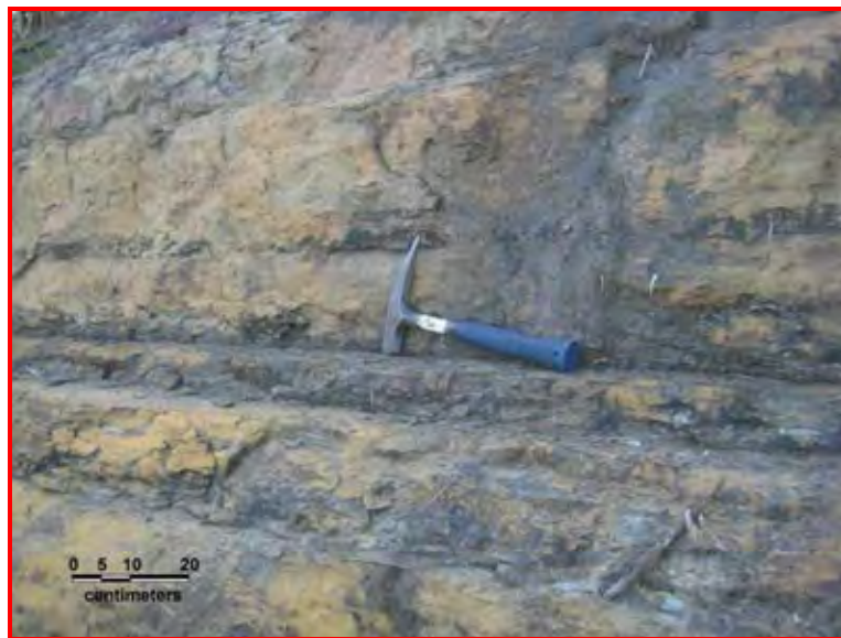
Figure 3.17 Shale exposure is approximately 6 meters high and 15 meters in width (looking south).
