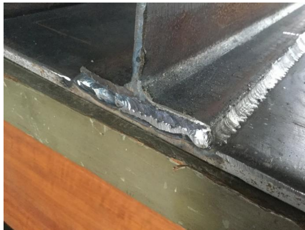
Figure 3.2 Welding between steel beam and cover plate.
