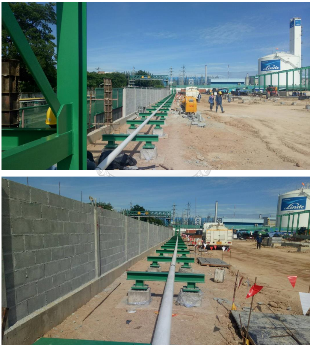
Figure 58 : Actual photos from the construction site
