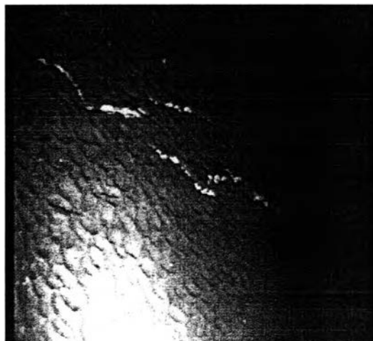
Figure 1.1 Scallops found on outlet feeder pipe k16 (Lister, 2004)
