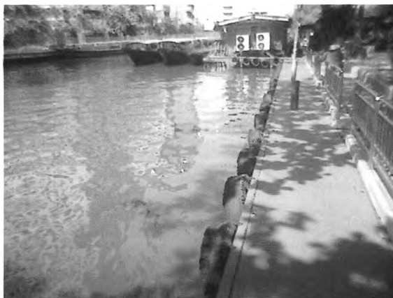
Figure E.4 S 4 , Wat Sri-boon-reung pier (The Saen-Saeb Canal)
