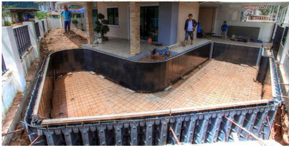
Figure 2-13 Vinyl liner structure
