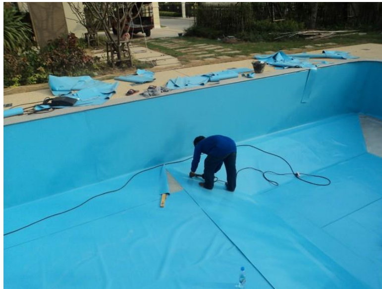
Figure 2-12 Vinyl liner installation
