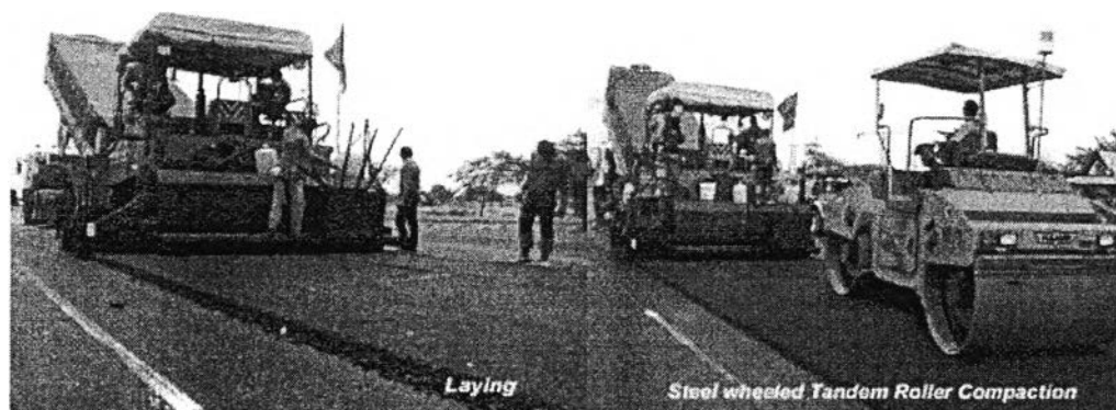
Figure 2.5 Laying and Steel wheeled Tandem roller compaction.
