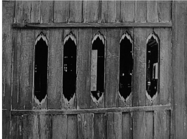
Figure 8. Detail showing the sliding panel type of window in Muang Pon Village, Mae Hong Son
