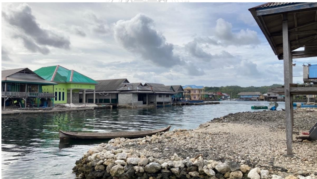
Figure 33. Reclamation of land from piling reef stones in the Mantigola Bajau (15 May 2021)
