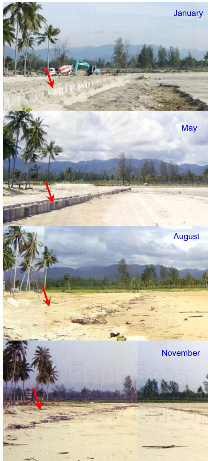
Figure 4.46 Comparing photographs of inlet/outlet mouth (looking south) at Blue Village Pakarang Resort showing deposition of sand in front of new sea wall. Deposition was clearly observed at concrete pipe (red arrow).
