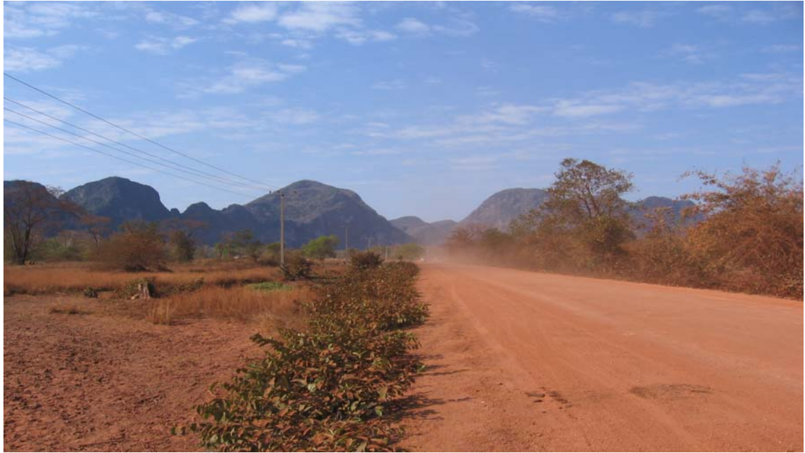
Figure 10: An example of the roads surrounding Route 9
