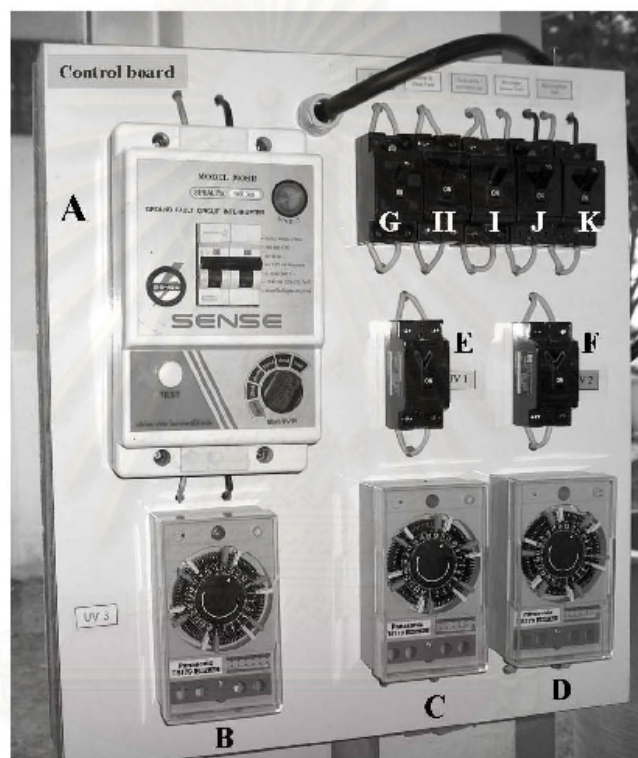
Figure 5.3 Control panel for continuous culture system of Figure 5.1, where:
