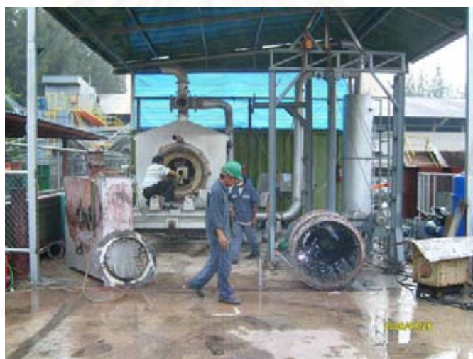
Figure A-16 Reparation of pilot-scale rotary cement kiln
