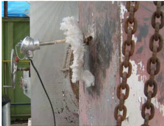
Figure A-13 Thermocouple in the inlet part of the pilot-scale rotary cement kiln
