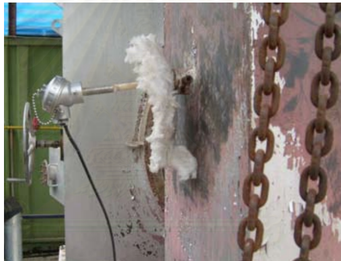
Figure 4.6: Thermocouple at the inlet part of the pilot-scale rotary cement kiln
