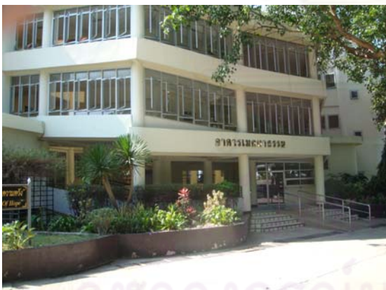
“Akhan Mettatham”: The hospital ward building to care for AIDS patients who are in less serious condition.
