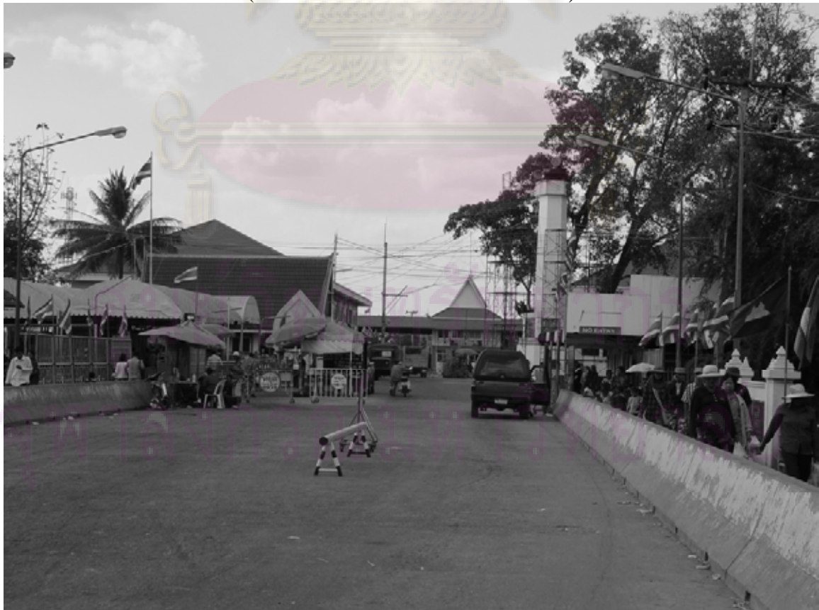
Figure 3.23 Bridge of the Two Countries: The inscription on this new bridge said that it was built in 1993 by Thailand, and donated by Britain as ‘a gift to the people of Cambodia’. In fact, benefits almost go ‘as a gift’ to the Thai side. (Photo taken on 27 December 2007)
