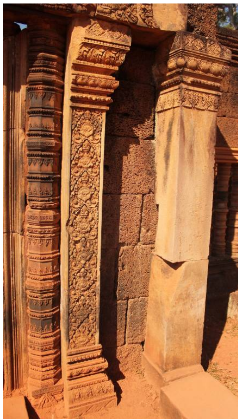
Figure 4.2 The fourth enclosure, east gopura , column, pilaster, pillar (from left to right)
