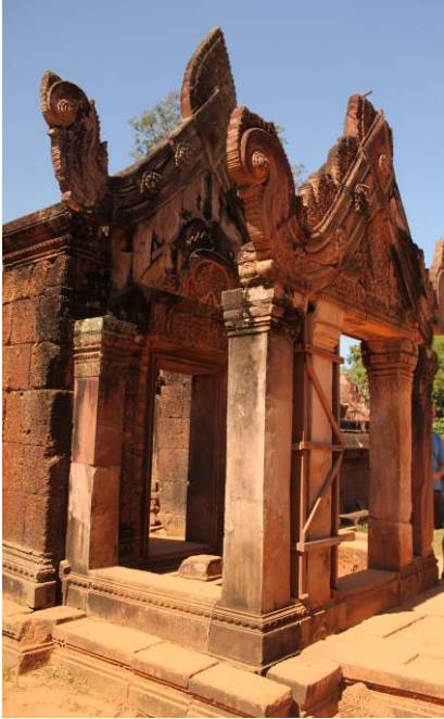
Figure 4.11 East Gopura II, triangular pediment
