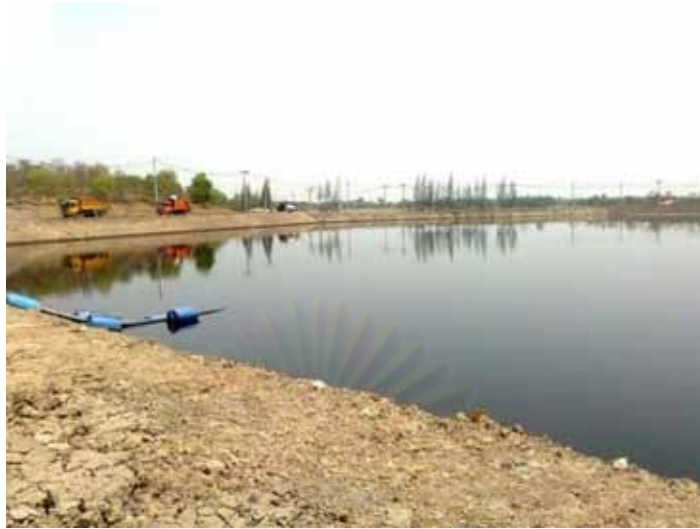
Figure A-1 Stabilized pond
