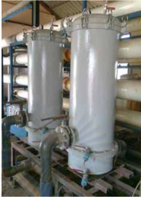
Figure A-5 Microfiltration (5 \mu\text{m} ) unit
