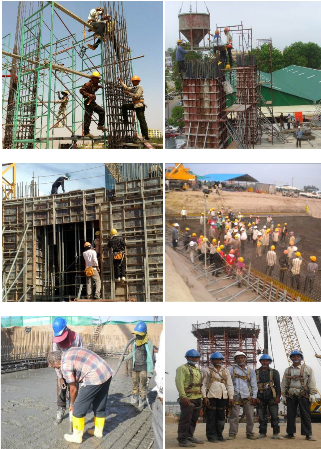
Figure 4.13 Site observation of worker using PPE (international contractors)
