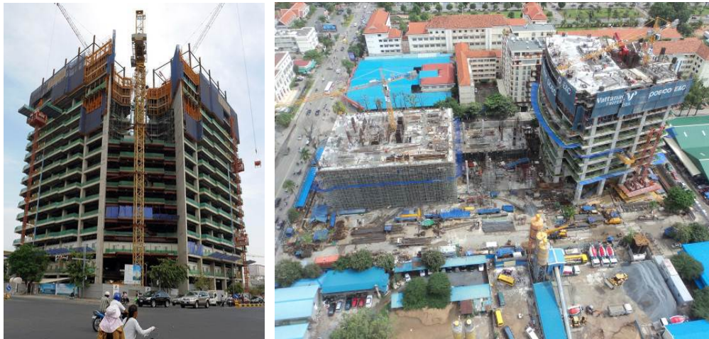
Figure 4.5 Gold Tower 42 & Vattanak project under construction in Phnom Penh
