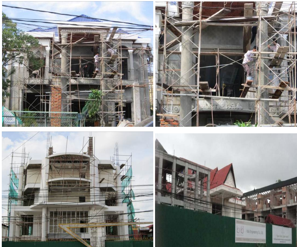
Figure 4.8 Building projects (under construction) in Siem Reap
