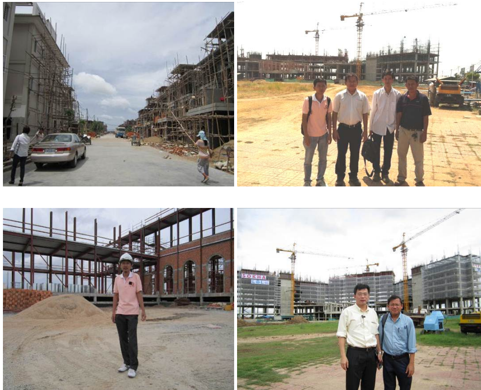
Figure 4.6 Building projects (under construction) in Phnom Penh
