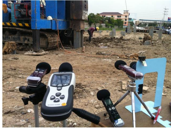
Figure 4.7 Experimental of noise hazard assessment system in construction site
