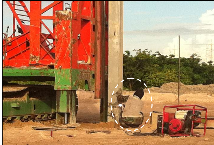
Figure 6.2 Labourers operating near generator in welding process
