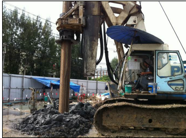
Machine operator in drilling work of bored piling operation
