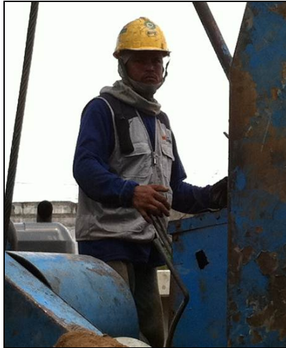
Attachment of instruments with construction workers
