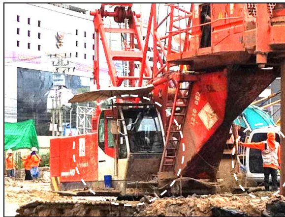
Figure 6.5 Current practices of operator and workers at some construction sites
