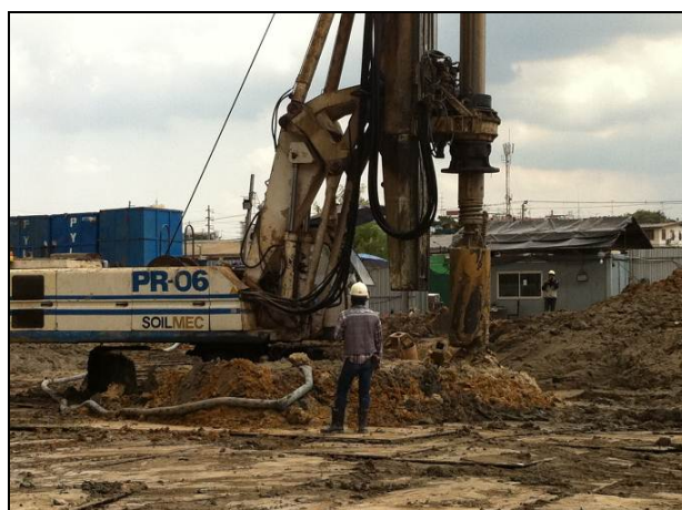
Foreman inspecting drilling work in bored piling operation
