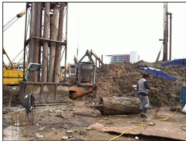
Labourer position near betonite storage during drilling work
