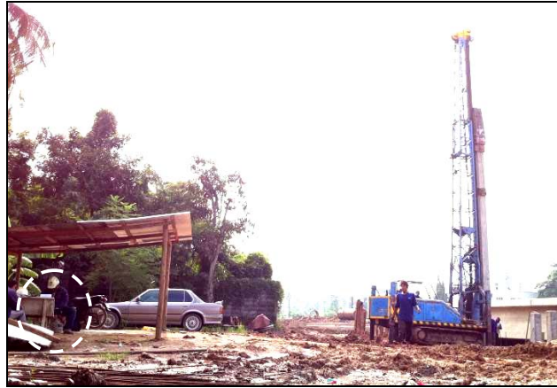
Figure 6.3 Position of foreman, labourer, operation in piling operation
