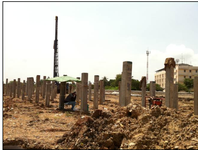
Position of foreman under shelter in drop hammer piling operation
