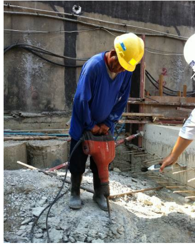
Figure 2.5 Jack hammering in construction site
