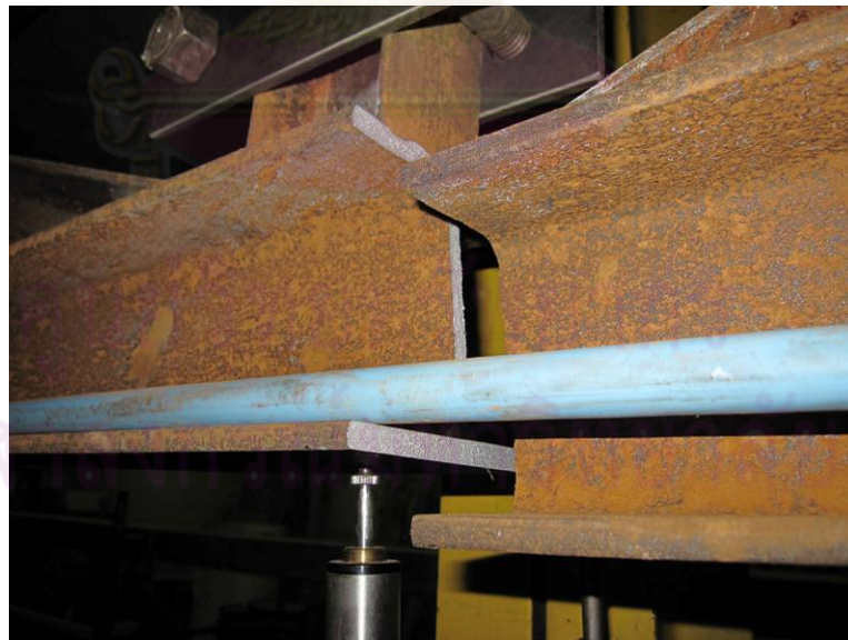
Figure 3.27 Complete fracture of the bottom chord of Specimen A4
