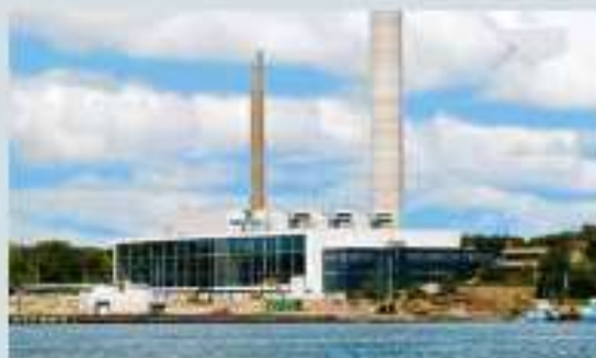
Coborg Energi AB, Rya, Gothenburg: Three 45MW(e) SGT-800 gas turbines at the combined heat and power plant provide electricity and heating to the city of Gothenburg.
