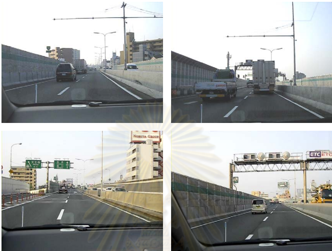
Figure 4-3 Ultrasonic Detector on Hanshin Expressway, Osaka, Japan
