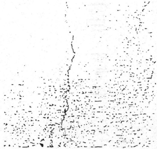
B. SHRINKAGE CRACK
