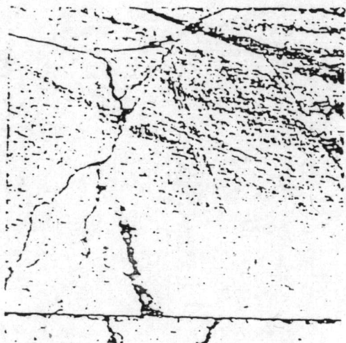
C. DIAGONAL CRACK
