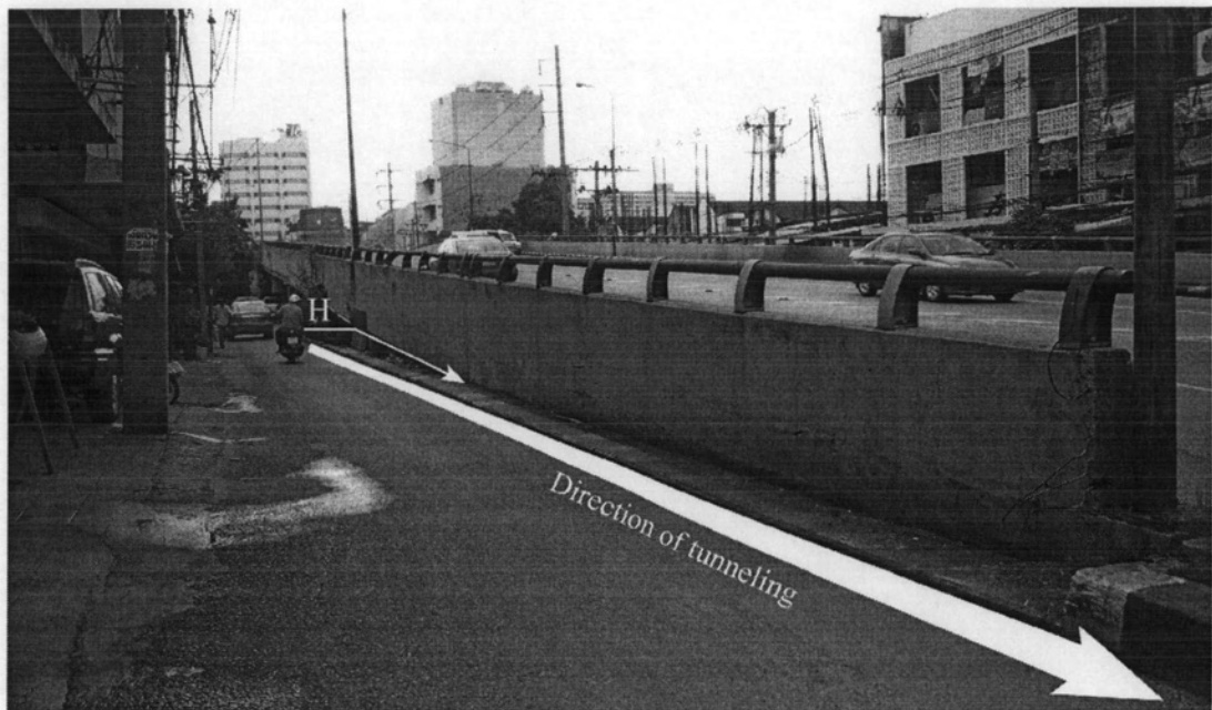
Figure 7.13 Location of point H monitored on Klongtan bridge
