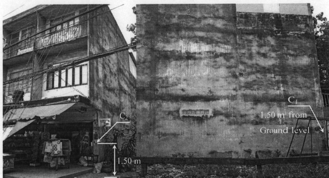
Figure 7.15 Location of point C_1 and C_2 monitored on 3-storey shophouse
