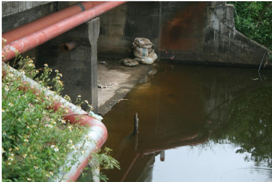
Figure G.2 The weir at Lake 2
