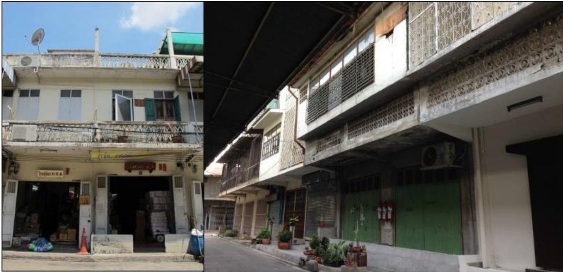
Figure 1.3 Expansion of shophouses in Thatien (taken by the author in 2014)
