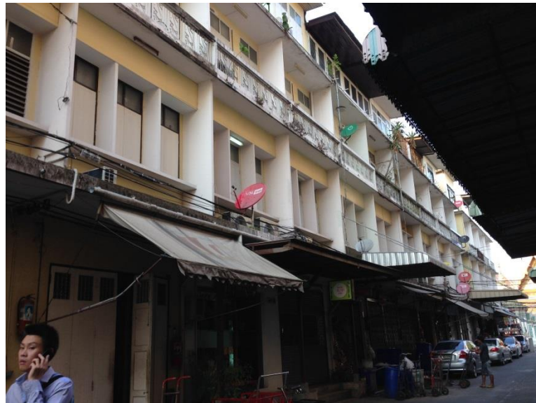
Figure 3. 46 Shelter and chamber above top floor provide more space.
