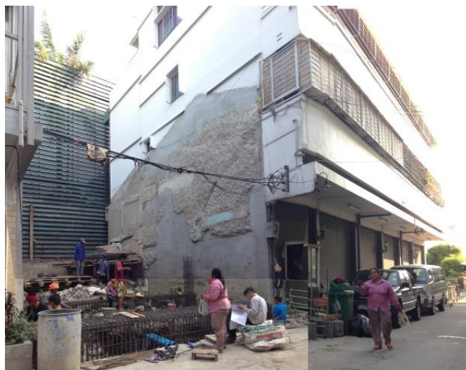
Figure 3. 45 New construction site in May 2014
