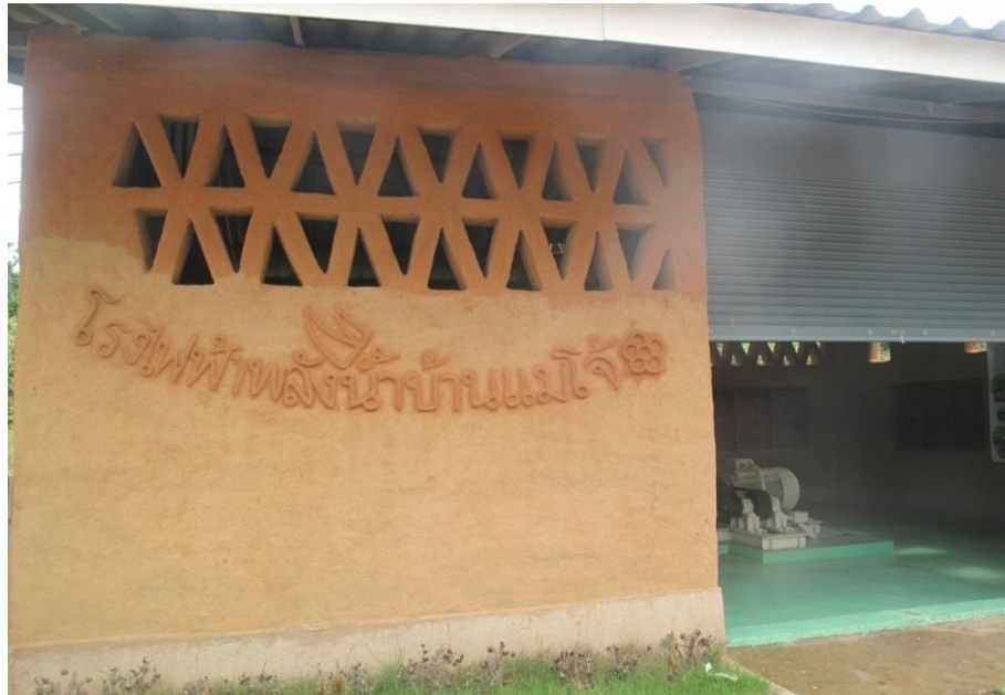
Figure 12 Mae Jo's Clay-House VSP's House of the Generator
