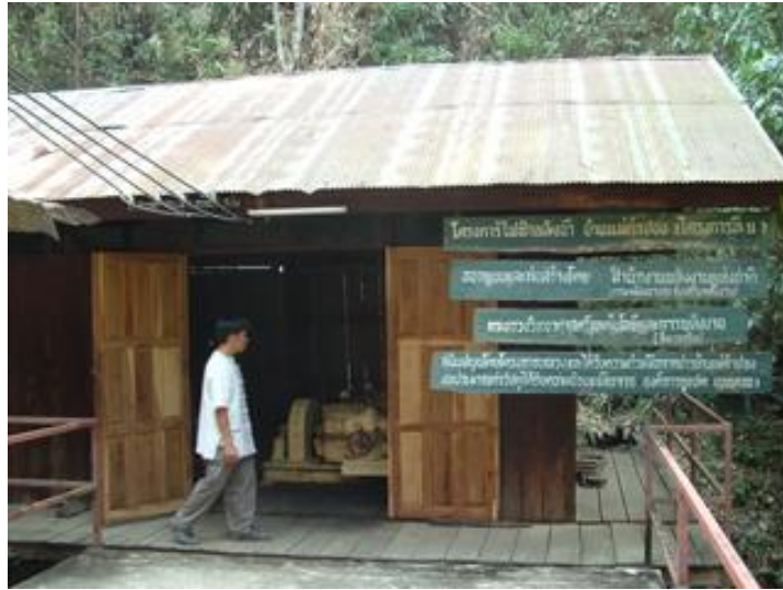
Figure 7 Mae Kam Pong's Off-Grid Power Generator
