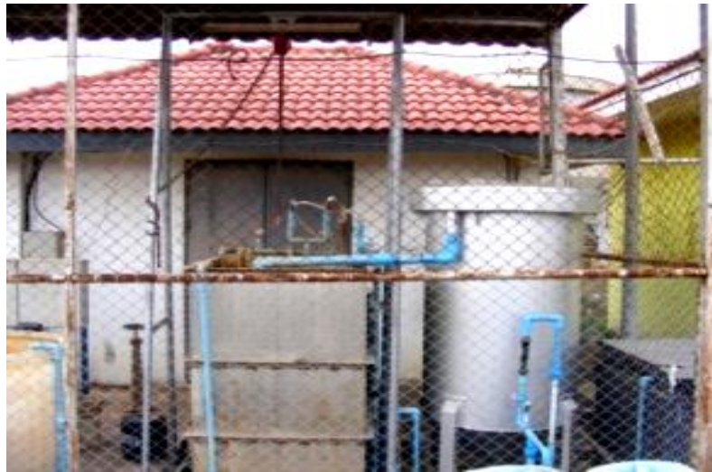
Figure A.1 Configuration of pilot-scale it-MBR at Nonthaburi disposal site, Thailand.
