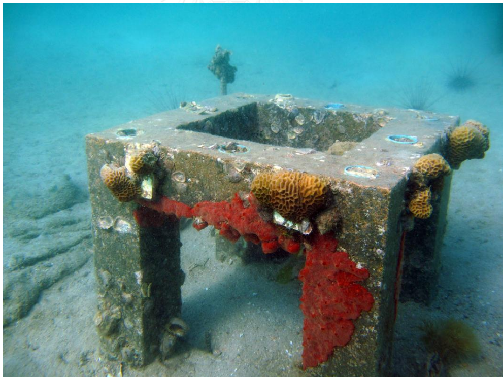
Figure 5- 3 Coral tiles attached on concrete block
