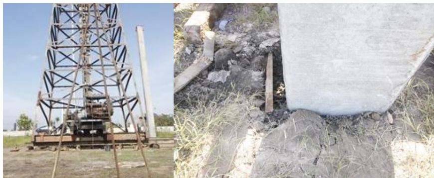
Figure 62 the effect of pile driving in site no. 2-2.
