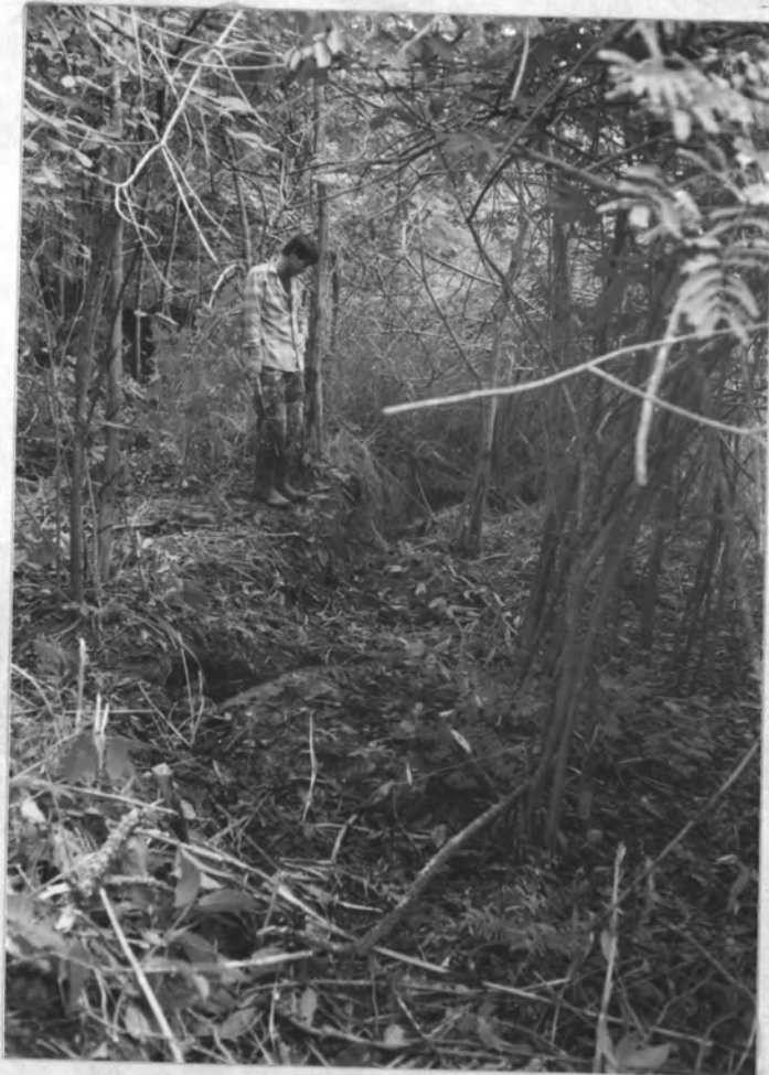
Figure 2.13 Progressive of tension cracks upslope.
