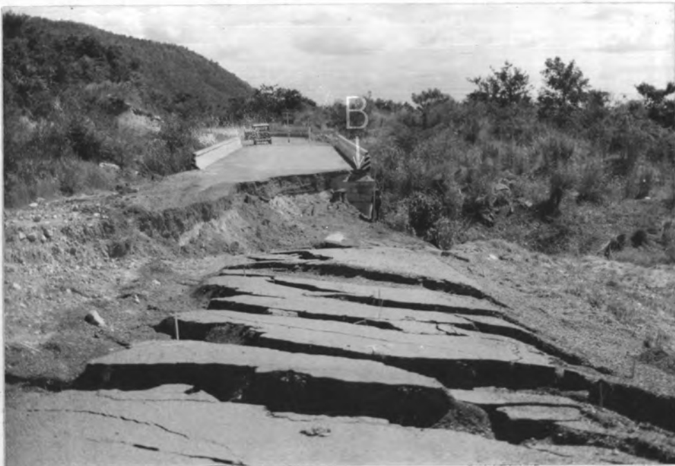
Figure 2.9 Vertical displacement at the major scarp, in 1986.
