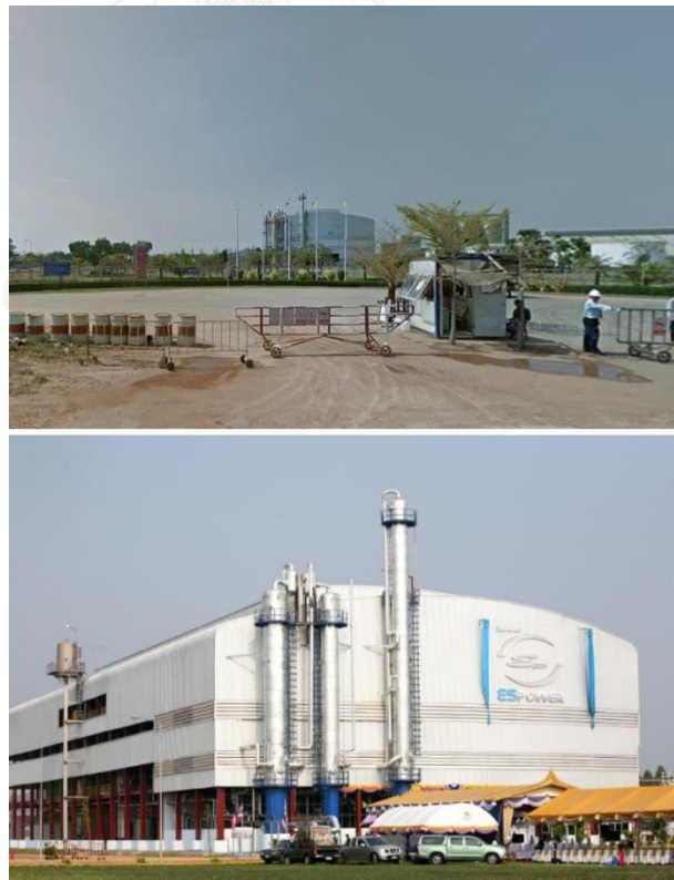
Figure 1. Eastern Sugar and Cane Company and ethanol plant
