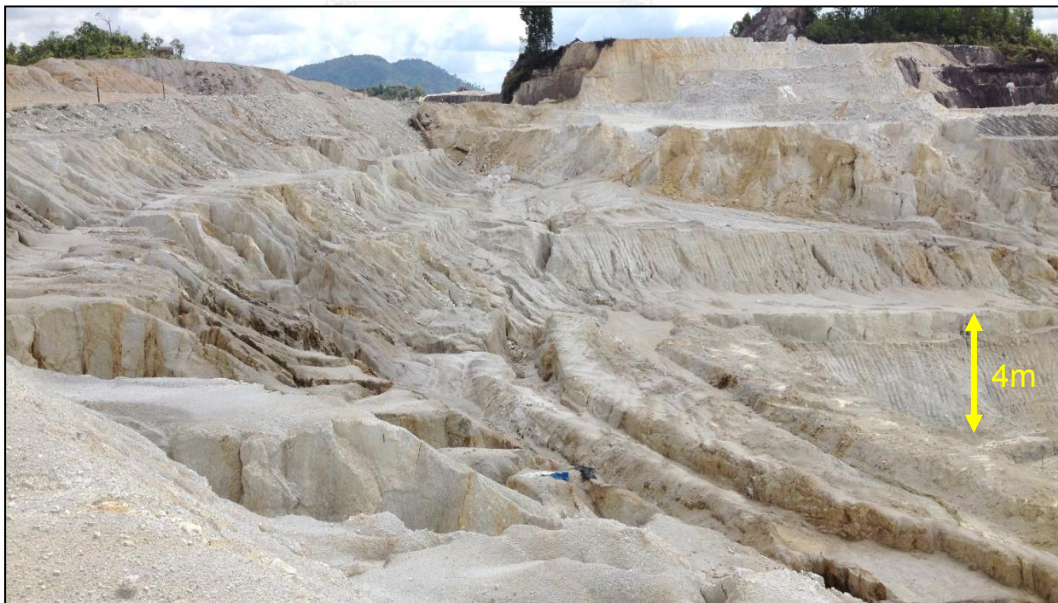
Figure 4. 2 Experience of erosional on kaolin slope due the affected from rain-flow.
