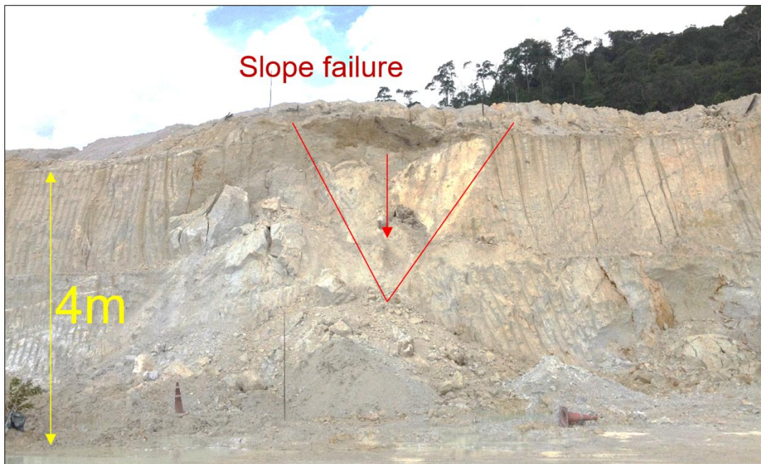
Figure 4. 1 Typical plane failure on kaolin slope at pit MF-2C. (May 2, 2015)
