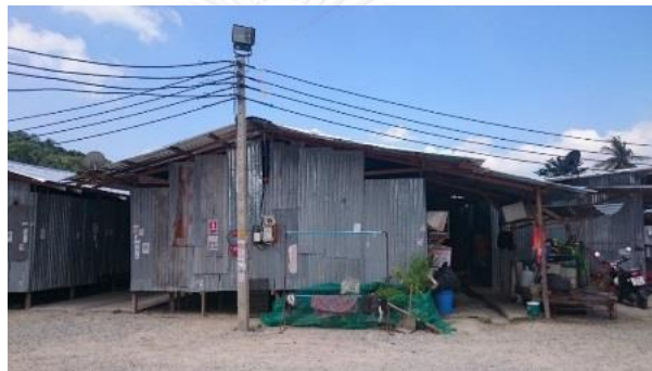
Figure 27. Univance New Factory Campsite, Pintong Industrial Park, Thai Kajima, 2015
