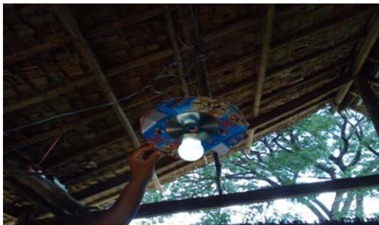
Picture 5.14 The use of CD to reflect the light from the bulb (Author's Photograph)
