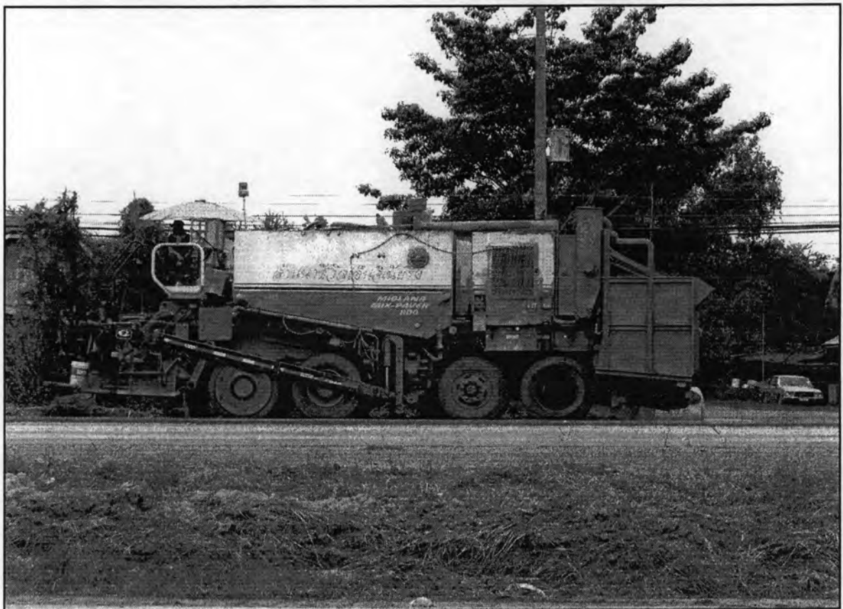
Figure 2.3 Mix and paver machines
