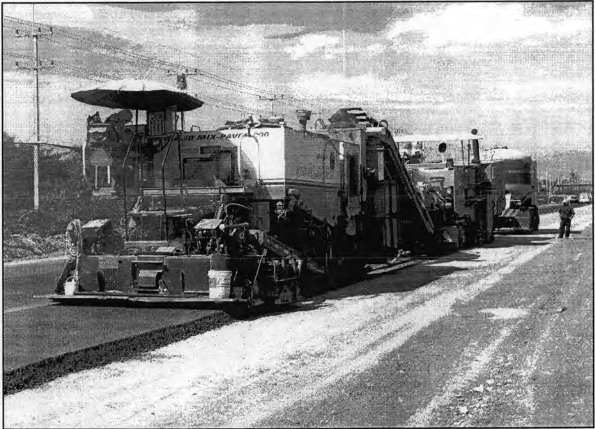
Figure 2.7 Paving modified RAP materials
