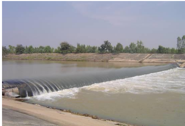
Figure 61 Ban-kae-wa weir (Photograph form Royal Irrigation Department).
