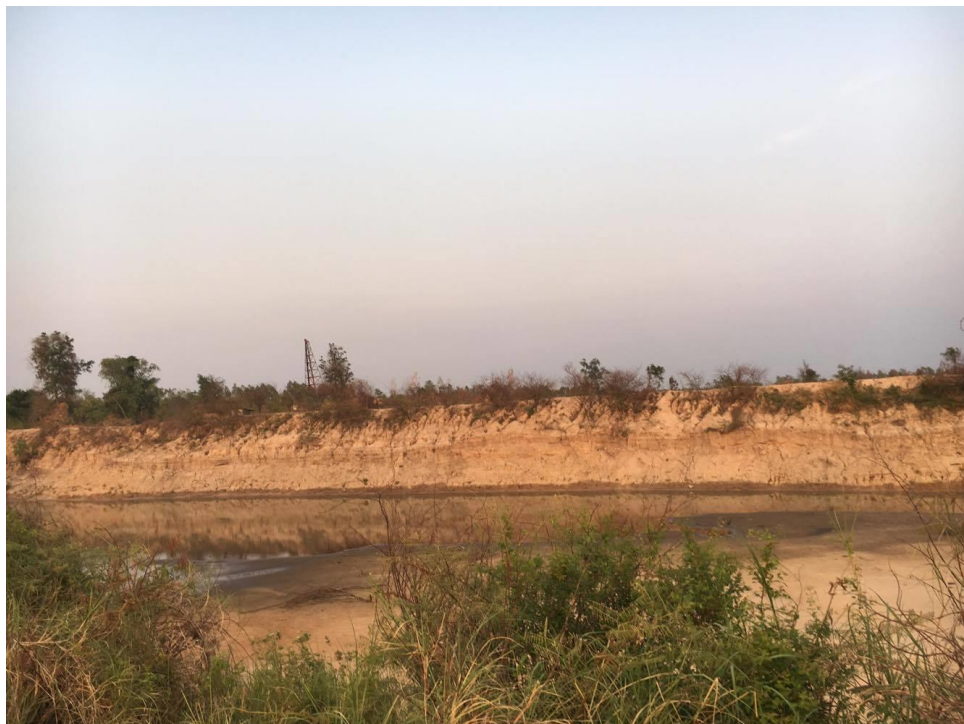
Figure 72 Bank profile location. This bank located opposite the GPR survey site no.1 in Mun River western part of Changwat Buriram, Thailand. From the top to the water level, the bank high is about 5 m.
