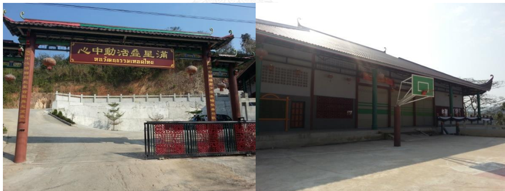
Figure 8: The Auditorium of Activity Center ( hui-guan ) in Ban Hin Taek village Source: This photo was taken by author on February 2017 at Ban Hin Taek village.
