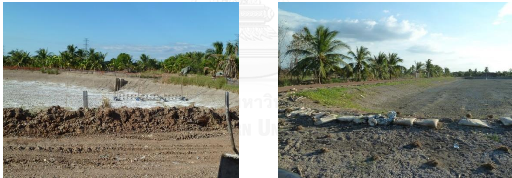
Figure 3.6 Action taken to prevent the damage from the worst flood in 2011
