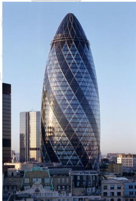
Figure 1.2 Swiss Re Building.
