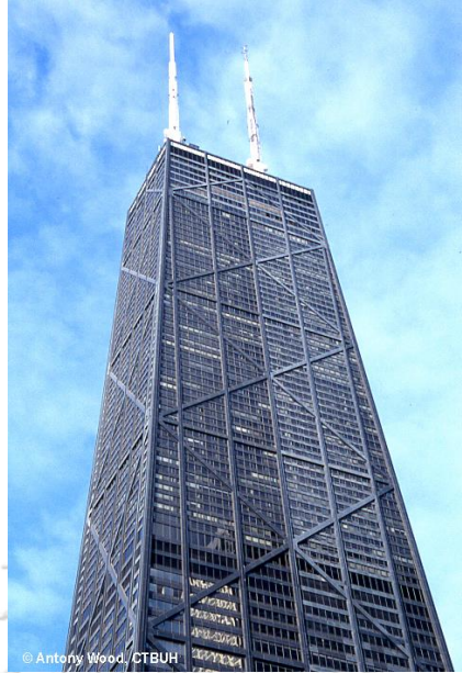
Figure 1.1 John Hancock Center.
